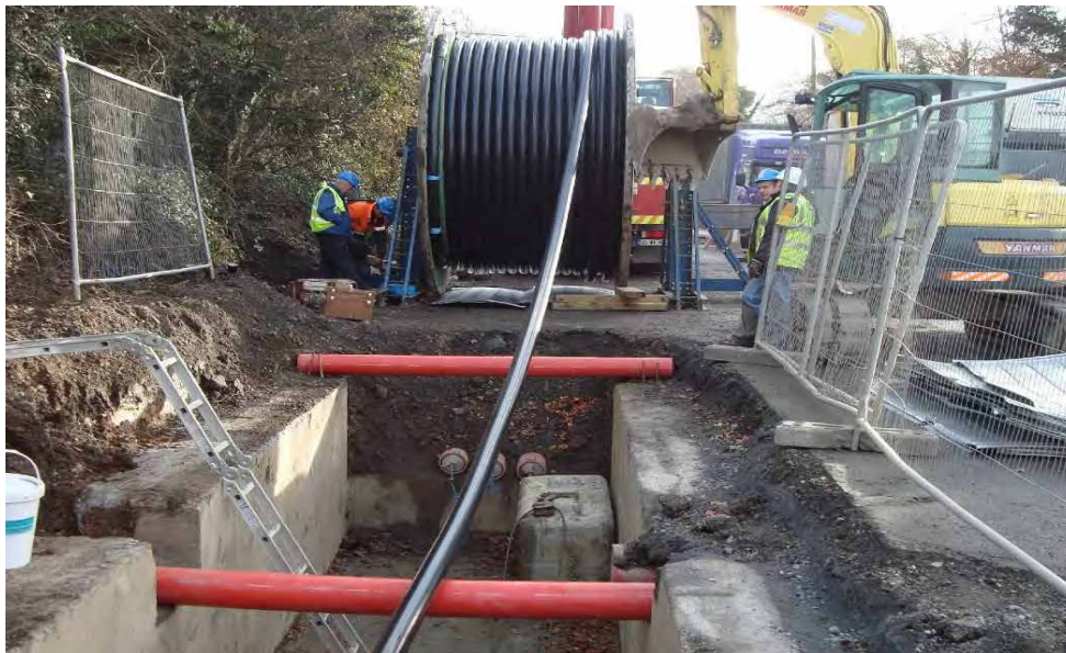
Figure 2-12: HV cable pulling procedure (Typical drum set-up)
