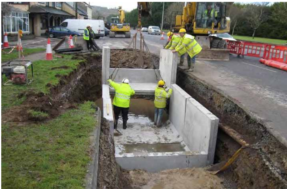
Figure 2-11: Typical joint bay under construction (pre-cast)
