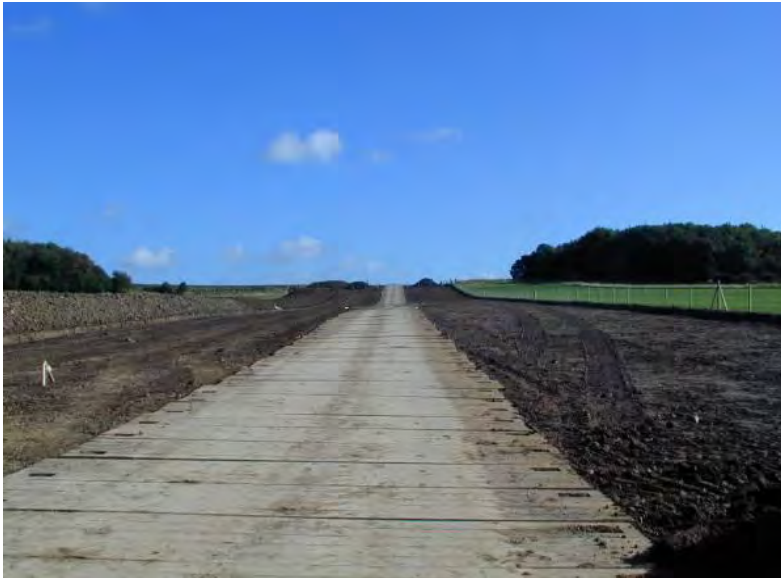
Figure 2-5: Cable Trench Preparation
