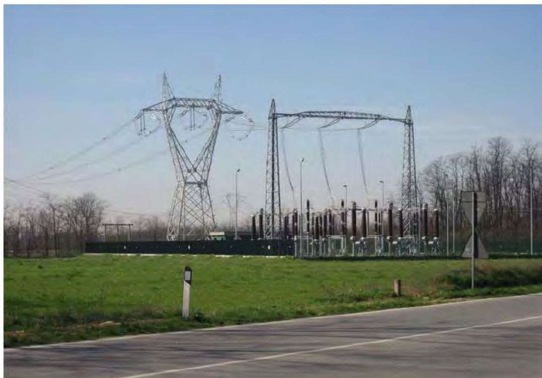
Figure 2-2: Typical Sealing End Compound
