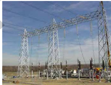
Figure 5: Overhead line cables transition station (400kV)
