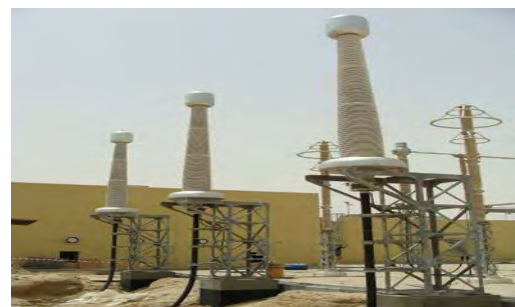
Figure 6: 400 kV Termination under construction
