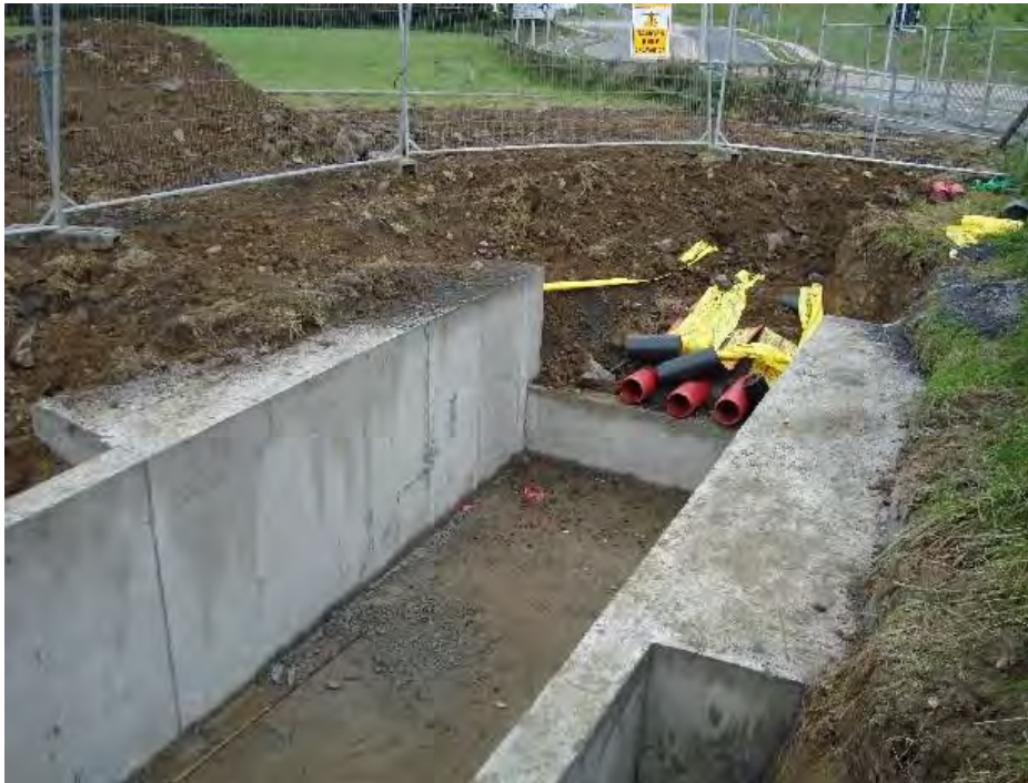
Figure 2-10: Completed joint bay prior to cable installation (in-situ)
