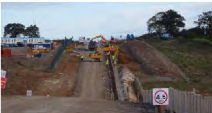
Figure 2-7: Cable Construction Vehicles
