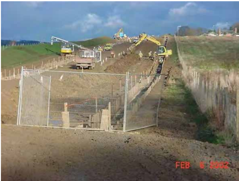
Figure 2-6: Cable Working Swathe for Construction
