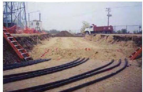
Figure 18: Installation of 400 kV XLPE cables
