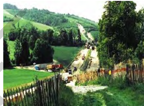
Figure 17 : cable route at site
